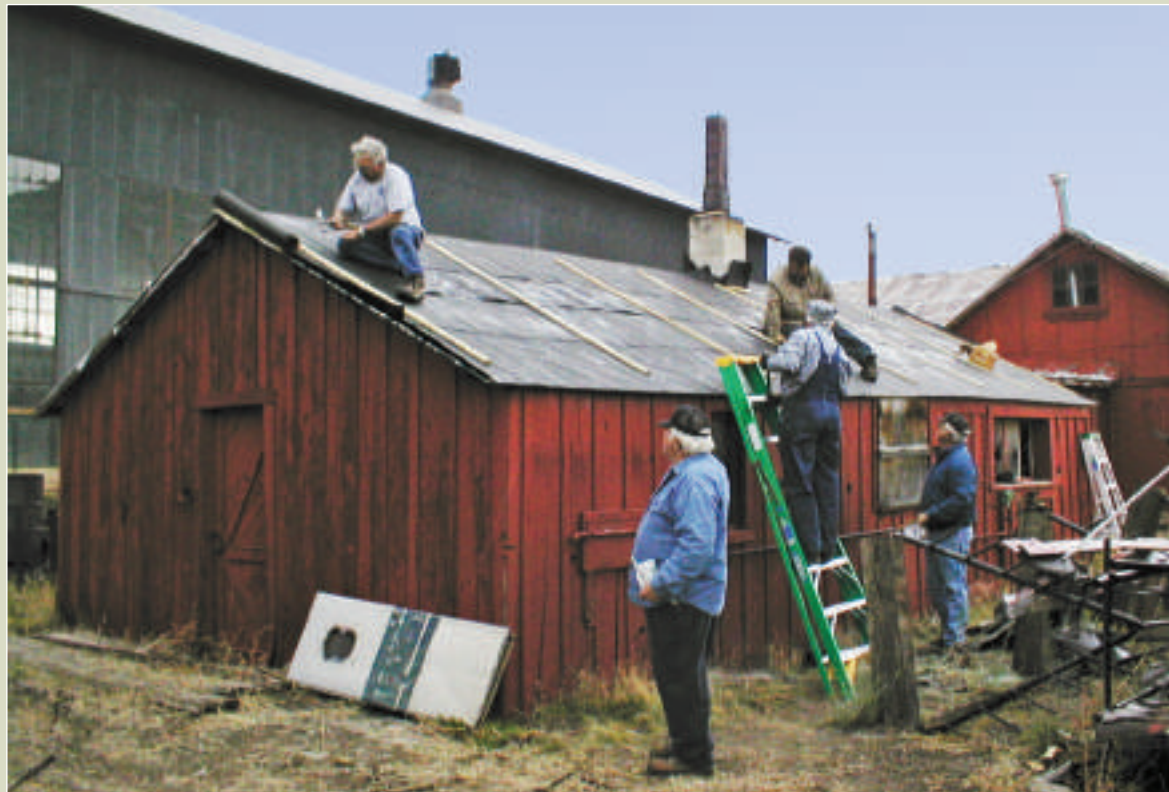
Volunteers repair the roof of one of the museum's 52 buildings.
